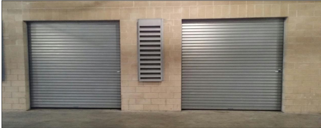
Insulated steel shutters when installed to core – filled masonry
