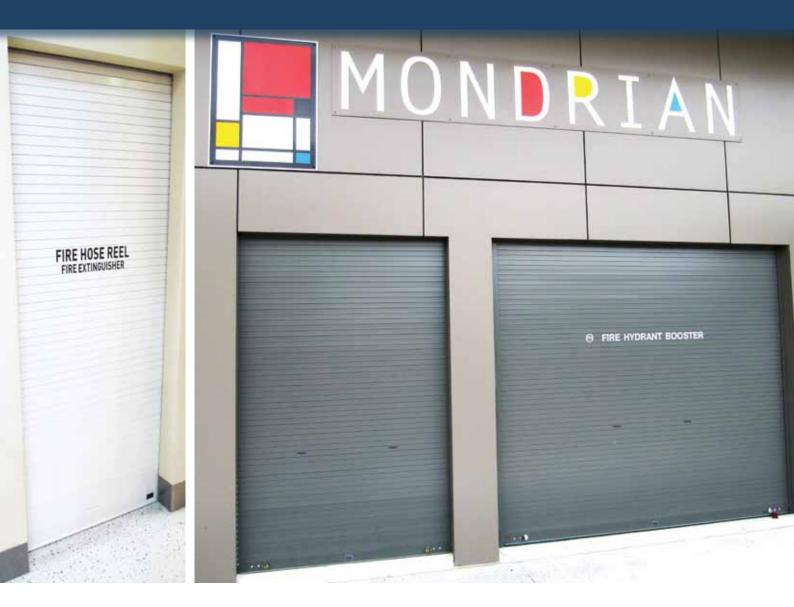
The Mirage Series 35 Mini Slat Roller Shutter has a small roll-up diameter and very easy operation due to the unique one-piece bracket and guide channel.
