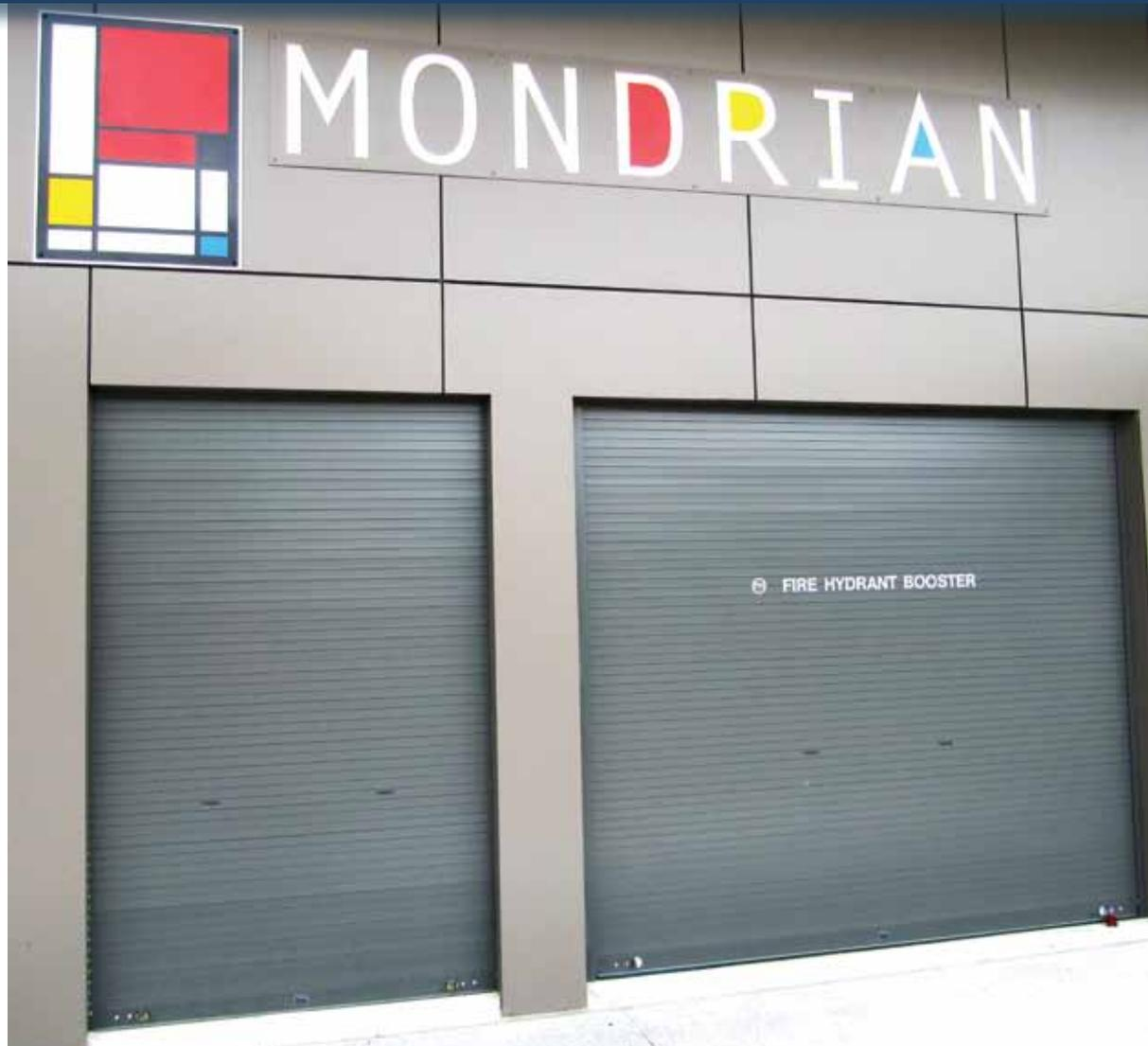
The Mirage Series 35 Mini Slat Roller Shutter has a small roll-up diameter and very easy operation due to the unique one-piece bracket and guide channel.
